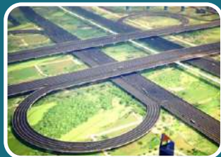
250 Mtr. wide 6 lane Ahmedabad-Dholera Express Way
