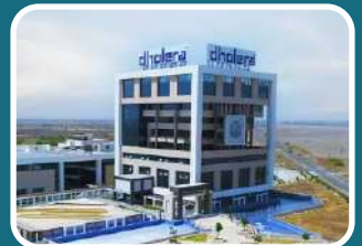
Dholera ABCD Building
